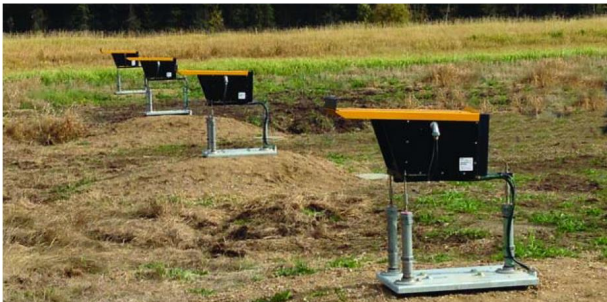
LED Single unit PAPIs with integral monitoring
