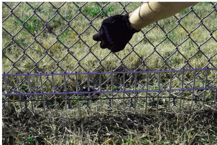
Figure 3-2 Fencing should also be trenched
