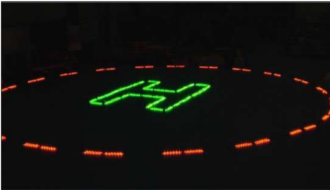
Figure 11-18. Helipad application of line lighting (source: CAA UK)
